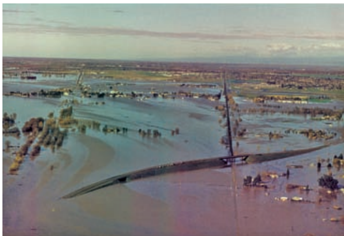
Urbanization on Central Valley floodplains increases risk to lives and property. Photo by Rand Schaal.
