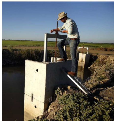
Photo: Liz Hafalia, The Chronicle Jacob Katz, California Trout senior scientist, opens a screw gate at rice fields in Woodland (Yolo County).
